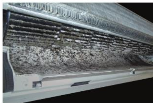
Mold thrives on mini-split blower wheels
